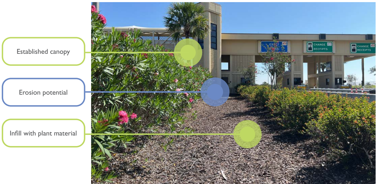
Image 5.2 SR 429 at New Independence Mainline Gantry
