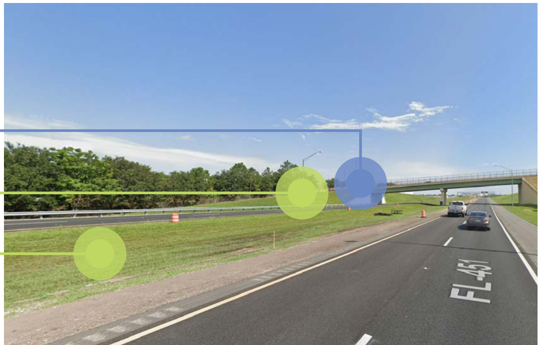
Image 6.8 SR 451 at John Rd
