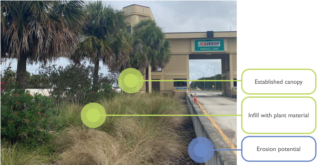
Image 5.1 SR 429 at New Independence Mainline Gantry
