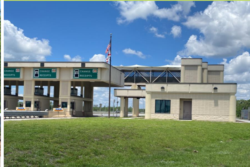
Toll Ramp Plazas and Mainline Toll Gantries
