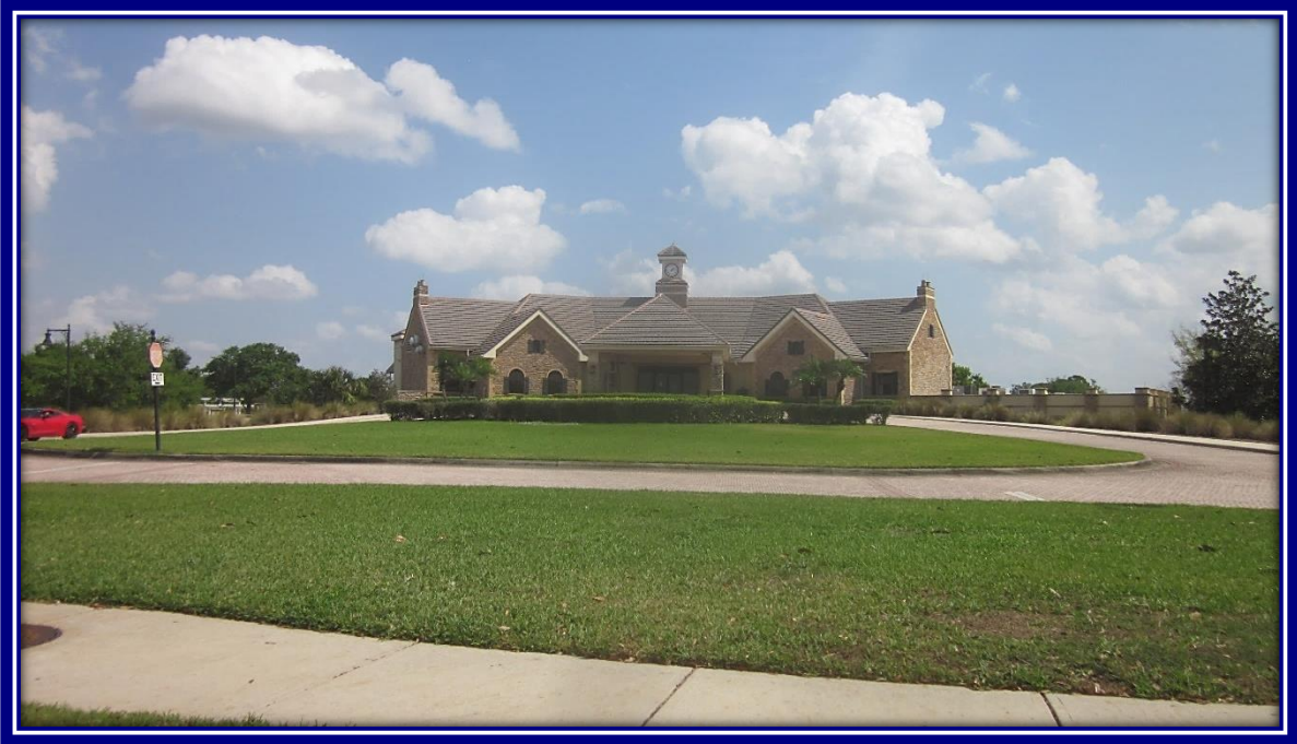
View of the Eagle Creek clubhouse. (Photo No. 3)
