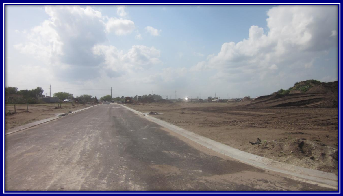
View of JK2B-2. (Photo No. 7)
