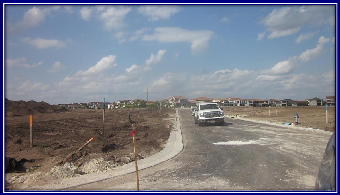
View of JK2B-2. (Photo No. 8)
